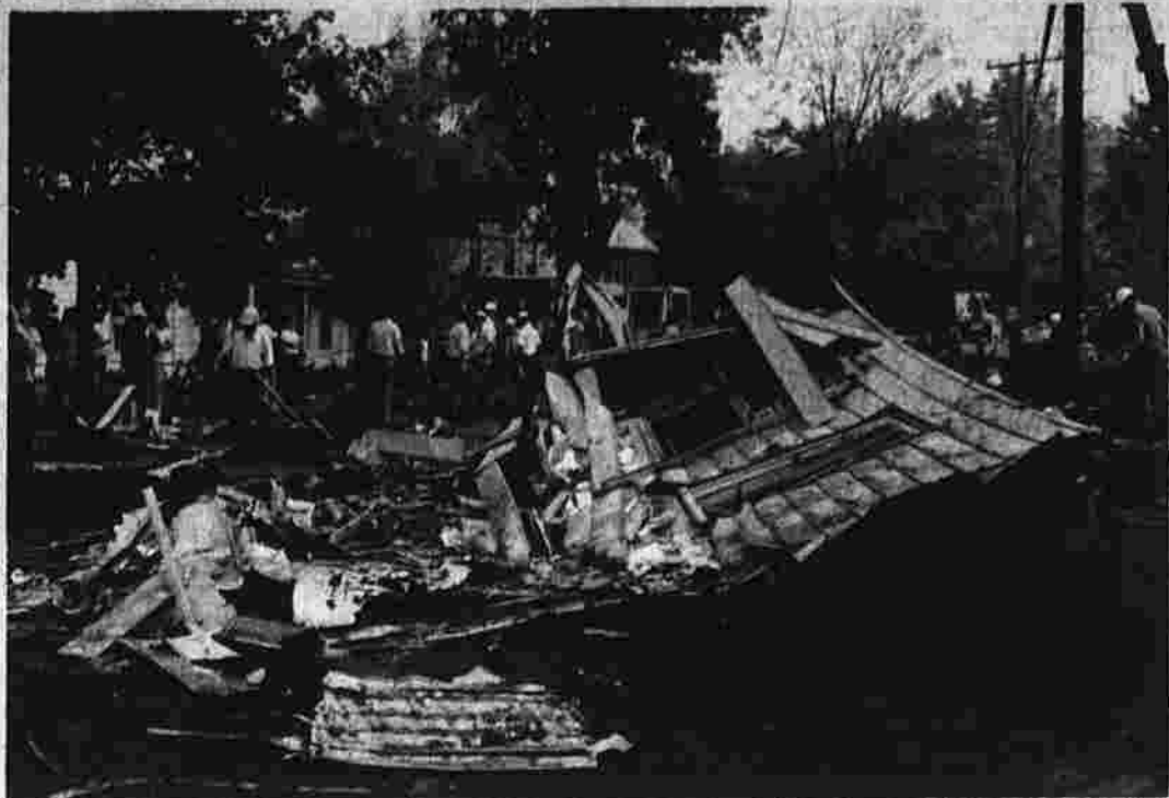
Wall blown out into roadway
